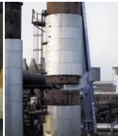
Demolition of steel structures
