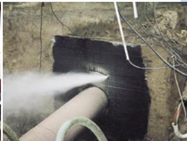
Cutting of reinforced concrete
