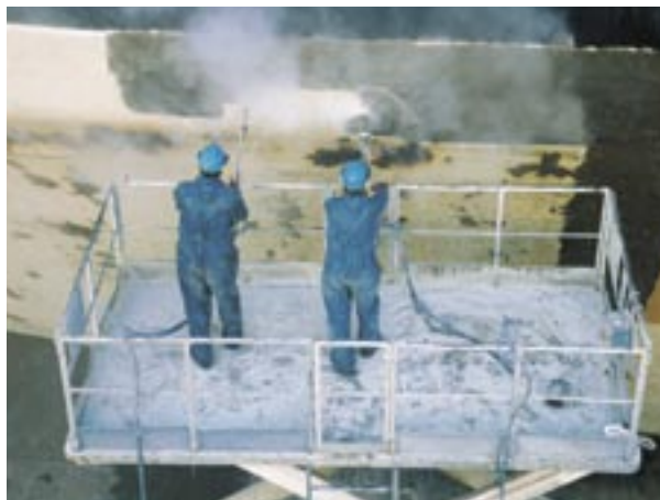
Surface preparation with two-gun operation
