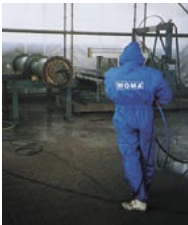
Cleaning of tube bundles
